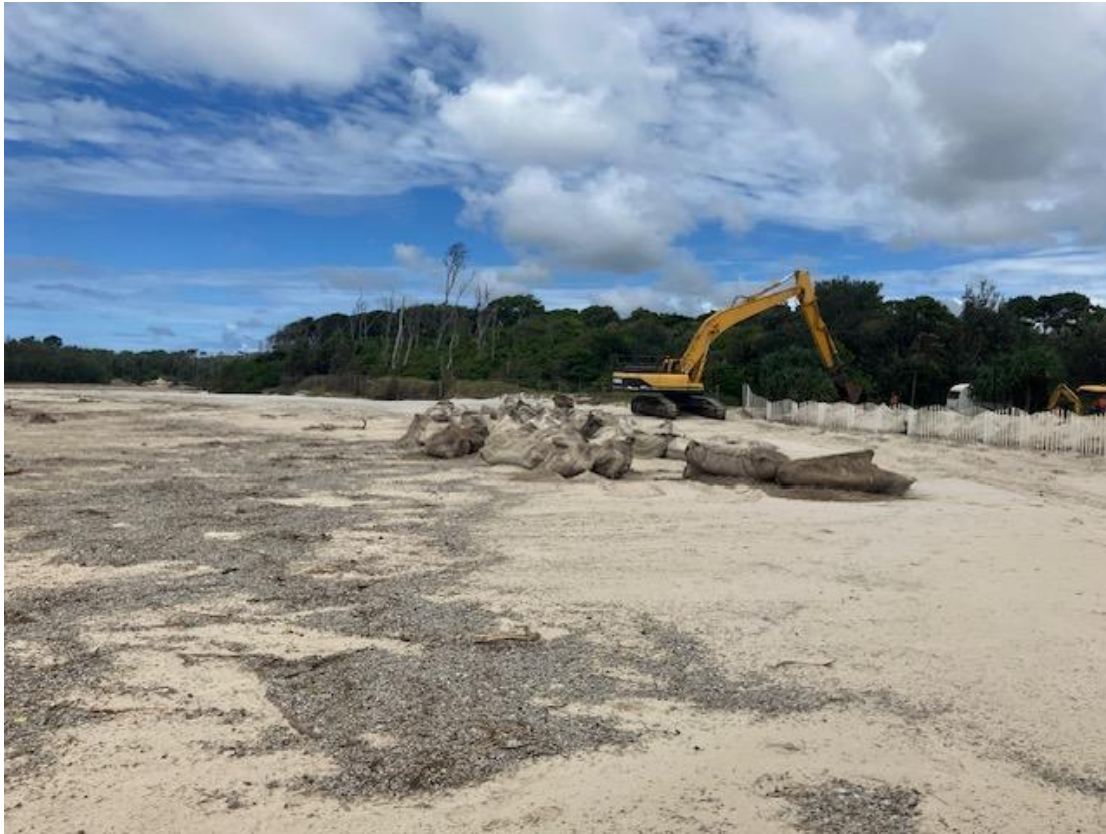
Figure 11: Repair works to the existing geobag wall (photo taken 12/03/25).
