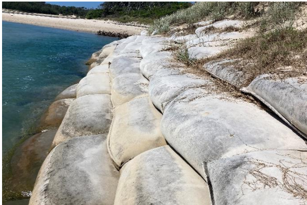
Figure 6: Existing geobag wall
