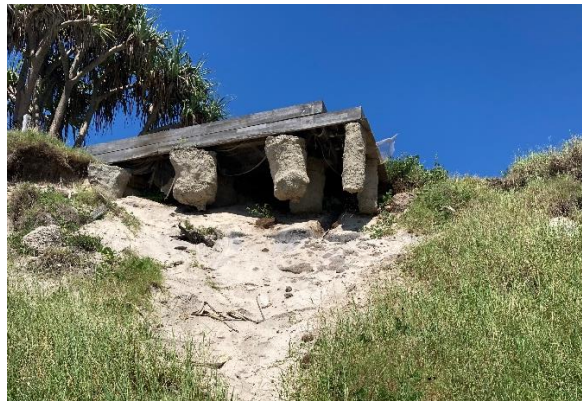
Figure 7: Viewing platform undermined by existing erosion
