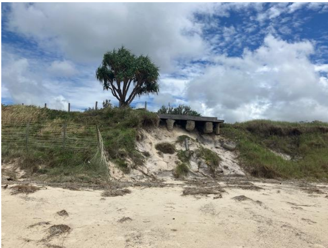
Figure 14: Western extent of geobag wall showing debris line from wave run-up during TC Alfred (photo taken 12/03/25).
