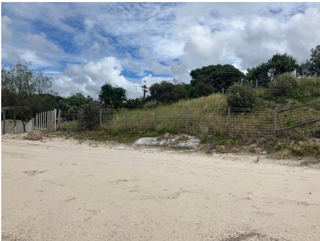
Figure 12: Sand accretion of the beach berm and part of the existing geobag wall. No wave run-up or debris noted from TC Alfred (photo taken 12/03/25).
